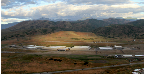
The Utah Data Center (UDC), a giant data storage facility in Utah, United States, used for mass digital surveillance purposes by U.S. intelligence agencies.
