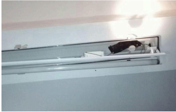
A microphone found inside a neon ceiling light in Modena, Italy, in December 2015 17 .
